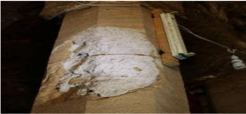
Fig. 7 Image showing damaged altar
