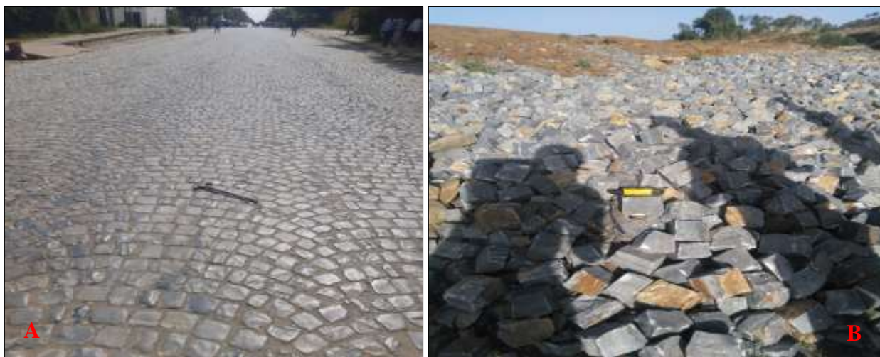
Figure 3: Figure A and B : (A) Cobblestone road pavement extending from Business College Adihaki branch to Adihaki secondary school, and (B) cobblestone blocks obtained from Shugala quarry
