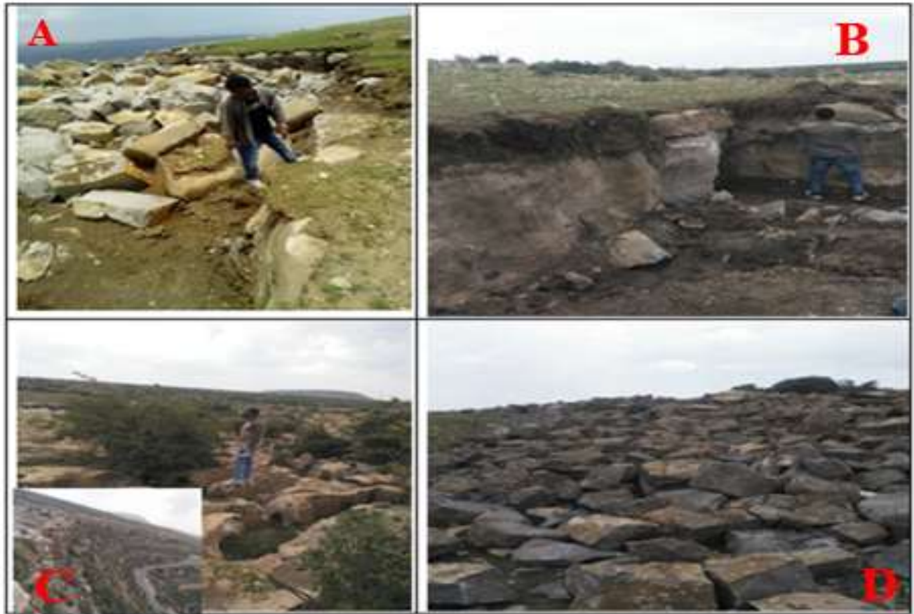
Figure 15: Figure 12: Illustrates the field exposure of the limestone units in the Mossobo area .(A) light-gray fossiliferous limestone (B), (C) Micritic limestone exposure with visible bedding planes and (D) Ligh-gray limestone exposure with polygonal joint patterns
