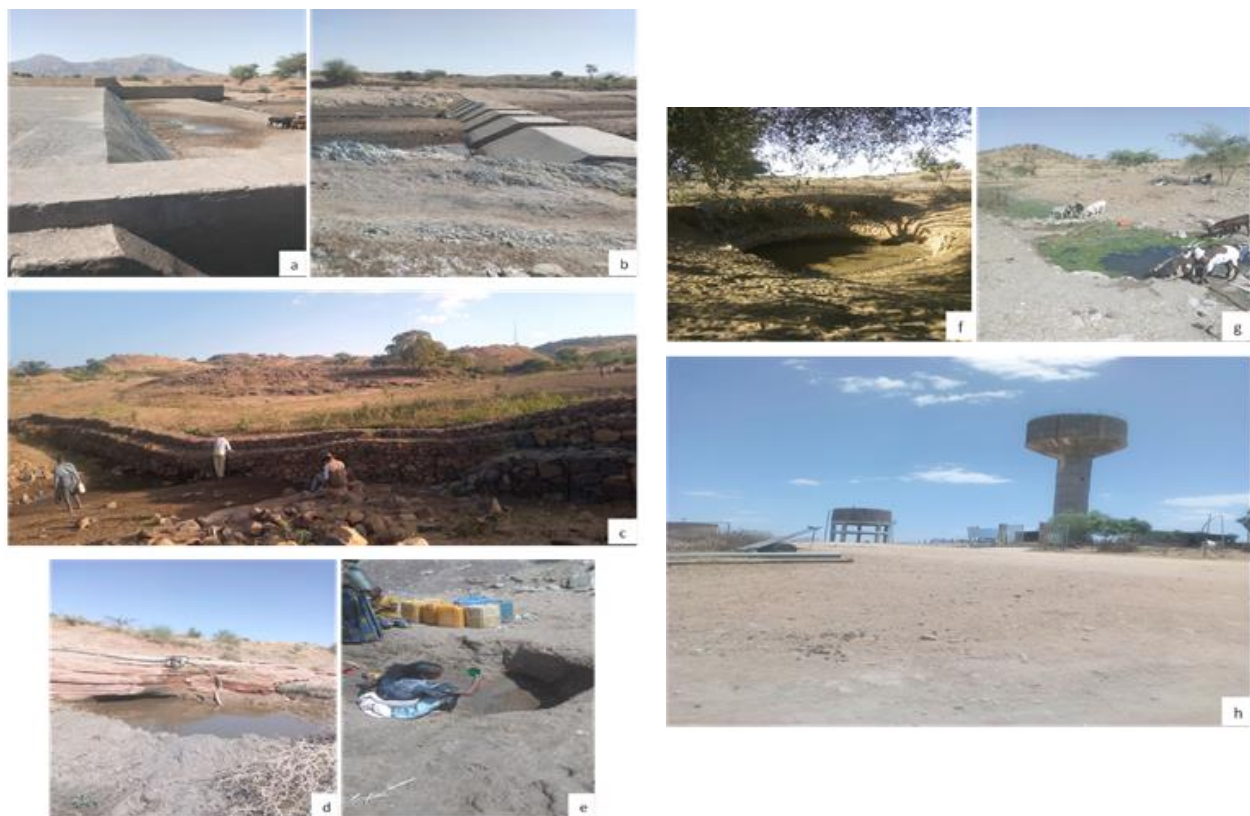
Figure 5.3: Some existed WH structures: (a) Concrete sand dam, (b) Concrete sand dam with multiple gates, (c) Gabion supported stone bund, (d) Pond motor pumping, (e) Hand boring in sand deposited stream bed, (f) Shallow open well, (g) Spring water at the metavolcanic rock, and (h) Water tanks used to collect water through pipe joining from surroundings for water supply to Yechila town; 250,000 m 3 (larger tank) and 100,000 m 3 (smaller tank)
