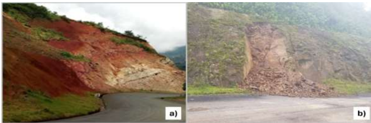
Figure 13: Middle trachyte flow exposures along the road. (a) With distinct paleosol horizon at Km 12+740, indicating ancient weathering surface; (b) Highly jointed and moderately weathered middle trachyte exposure at Km 63+460, showing slope face with potential for instability.
