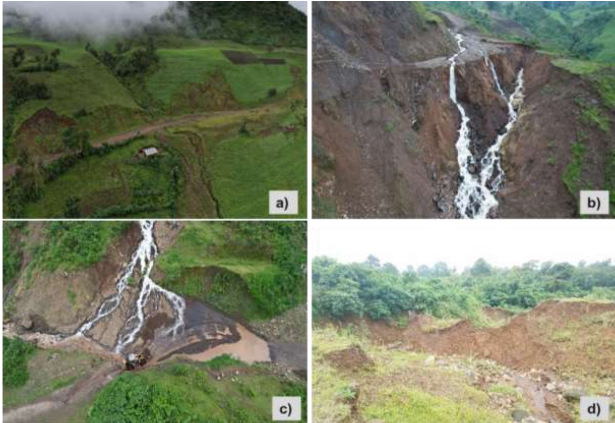
Figure 21: Typical examples of gully erosion. (a) and (b) Gully erosion damaging cultivated areas and causing deep erosion along the roadway near Washa; (c) and (d) widening and scouring around crossing structures near Tari and Mecha. (Photographs were taken in August 2021).
