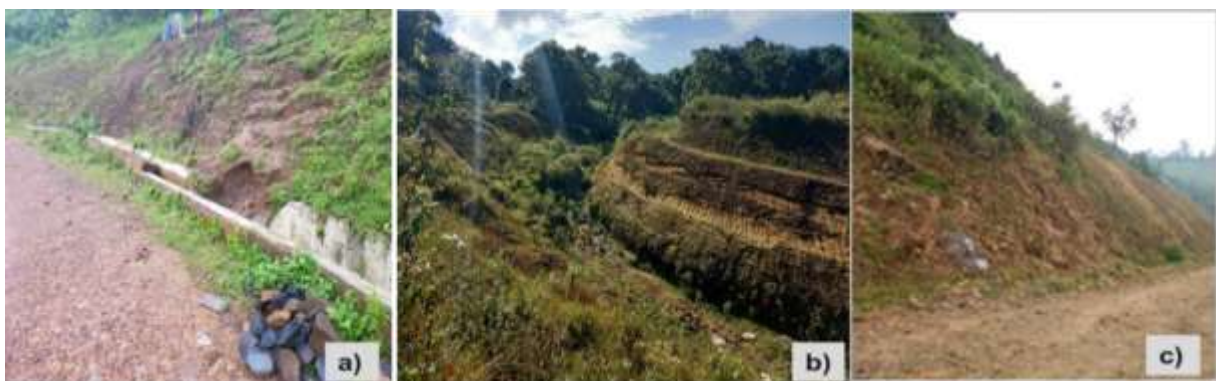
Figure 12: Photographs showing road cut exposures of upper trachyte flows at different locations: (a) completely weathered trachyte at Km 17+000, (b) highly weathered trachyte with deep box cut at Km 51+100, and (c) loose and weathered trachyte exposure with steep slope face at Km 65+500.
