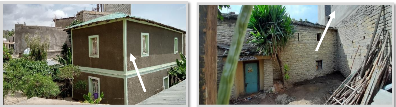
Picture 20: Impact of New Buildings in Kebele 010 (Left) and in Kebele 11 (Right). Field Survey, 2020.
