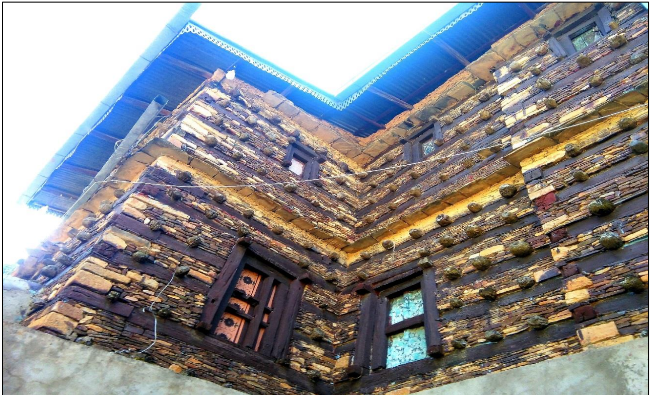
Picture 4: Tigray, Debre Damo Monastery, Monkey Head Wall Construction Technique. Field Survey, 2020.
