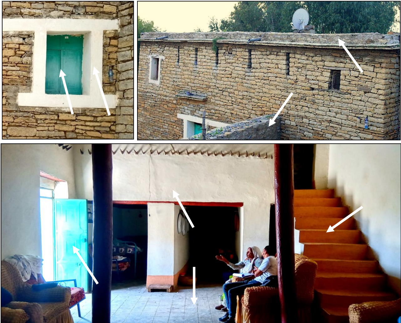
Picture 10: Resulted by Lack of Proper Maintenance and Qualified Expertise, the Mansion of Assefa Tedla (Compound one, Belay Assefa). Field Survey, 2020.
