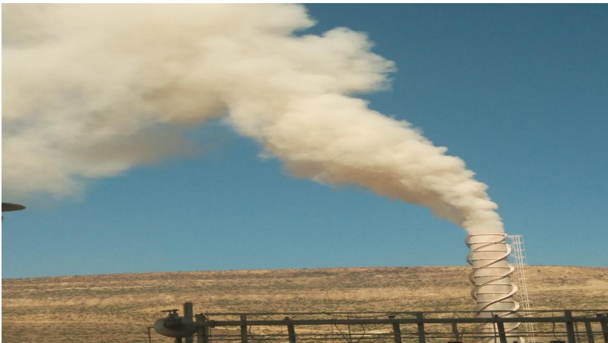
Figure 1: Line two raw mill excess chimney of MCF cement production
