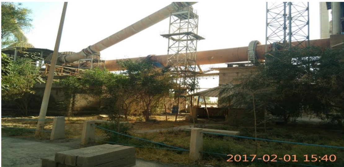
Figure 2: Kiln line two of MCF cement production
