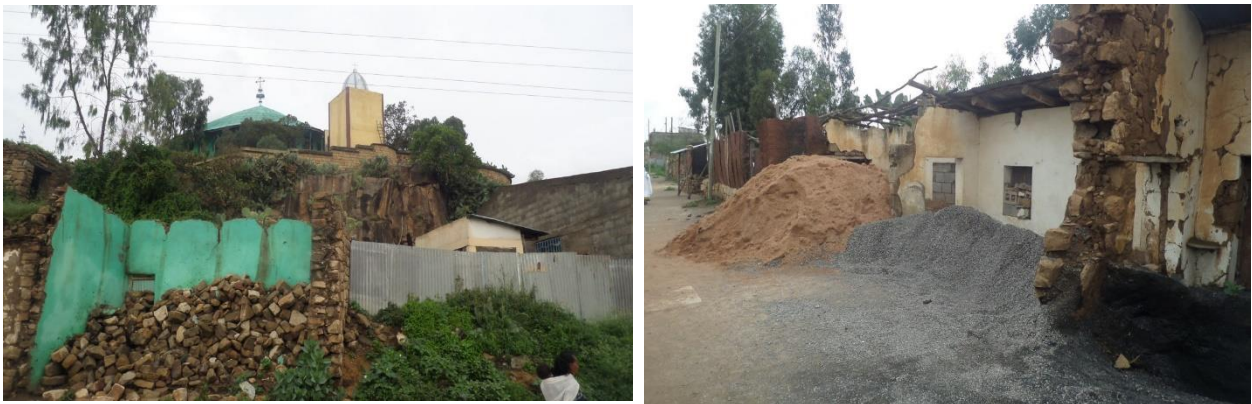
Figure 4. 5 Houses Demolished for Infrastructure Development
