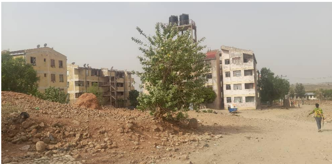
Figure 4-3. picture of the condominium housing
