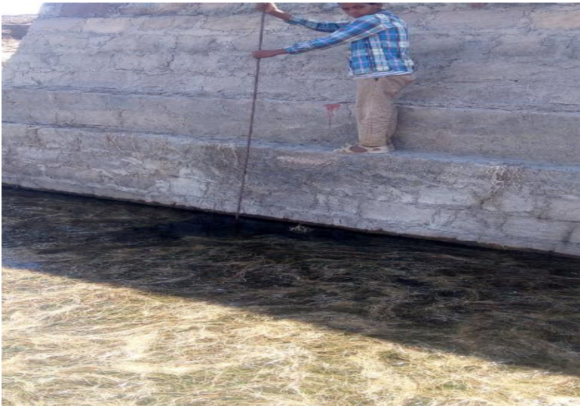
Figure 4. 2 daily measuring dam drawdown
