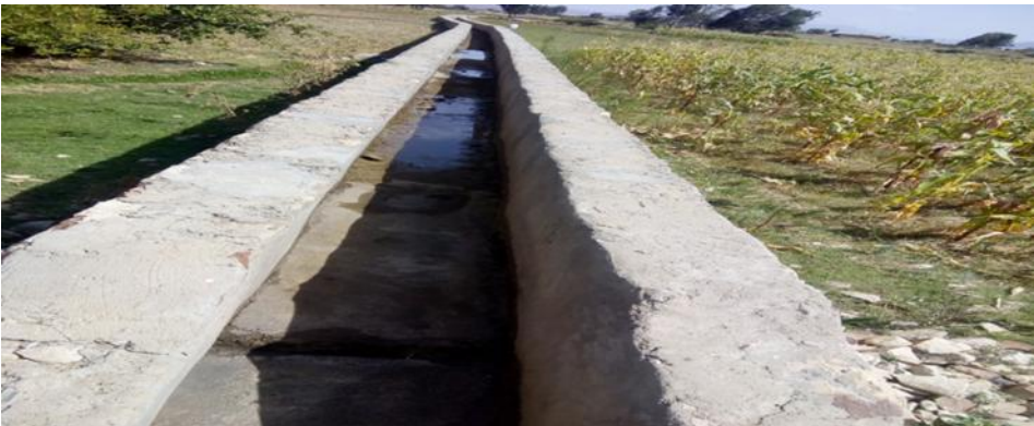
Figure 3. 7 Existed Lined Main Canal of Fre-lekatit irrigation scheme
